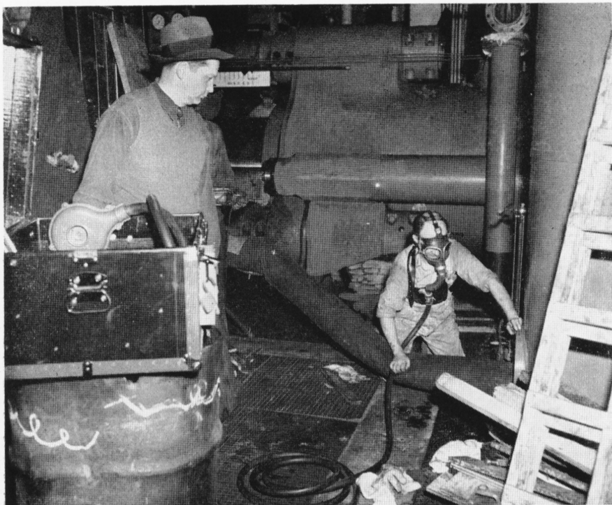
Harry Grover, inspector for Health and Sanitation Department, turns the blower on a line and mask, furnishing air to George Armour of the Paint Shop, who is about to enter a tank in the Extruded Rod Mill through an 11x15-inch opening. The Health and Sanitation men were called in on the job to supply fresh air to employees working inside a 6x15-foot tank.
